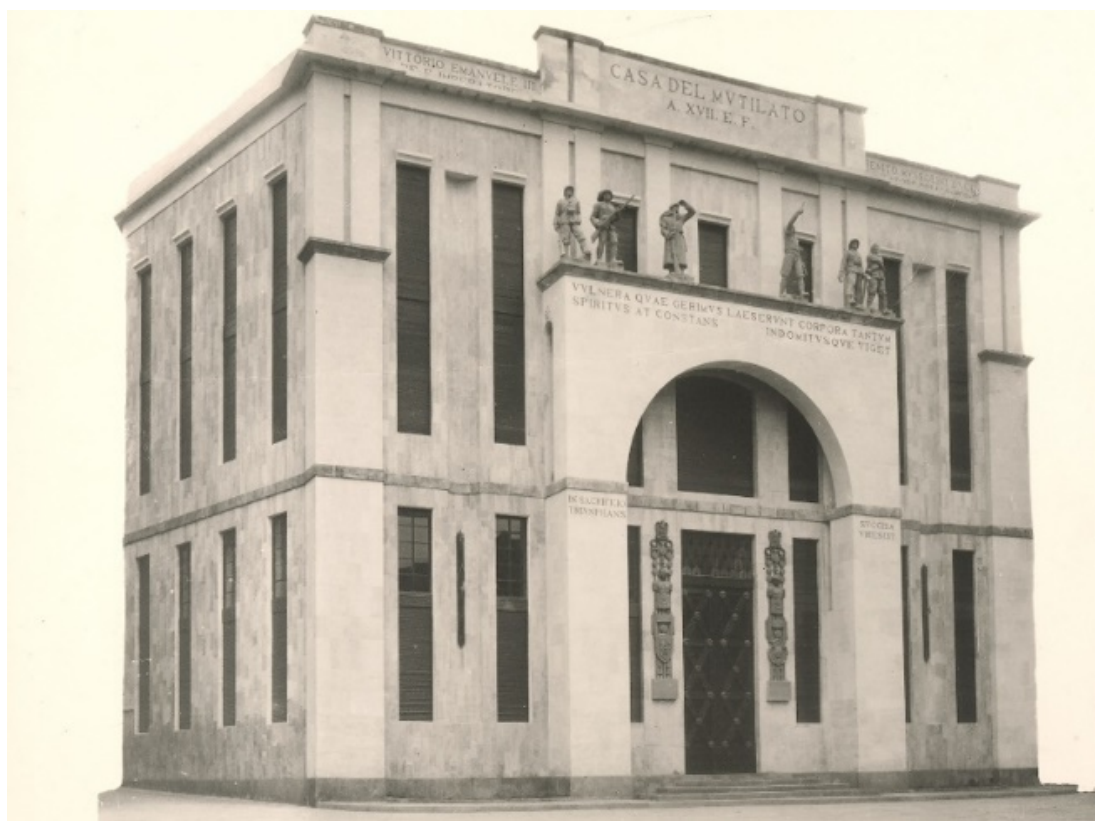
Figure 6: The Casa del Mutilato in Catania. Situation of 1939.
